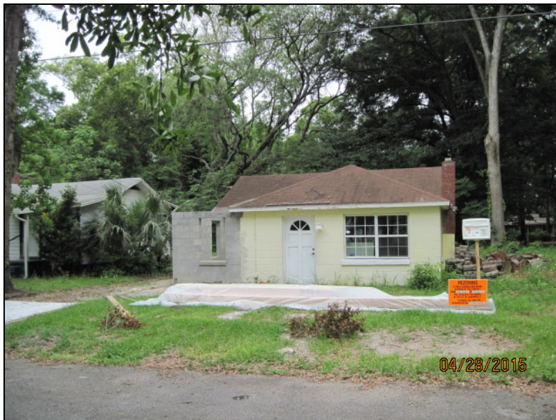
Single-family home for clergy, 4723 Pinedale Avenue
