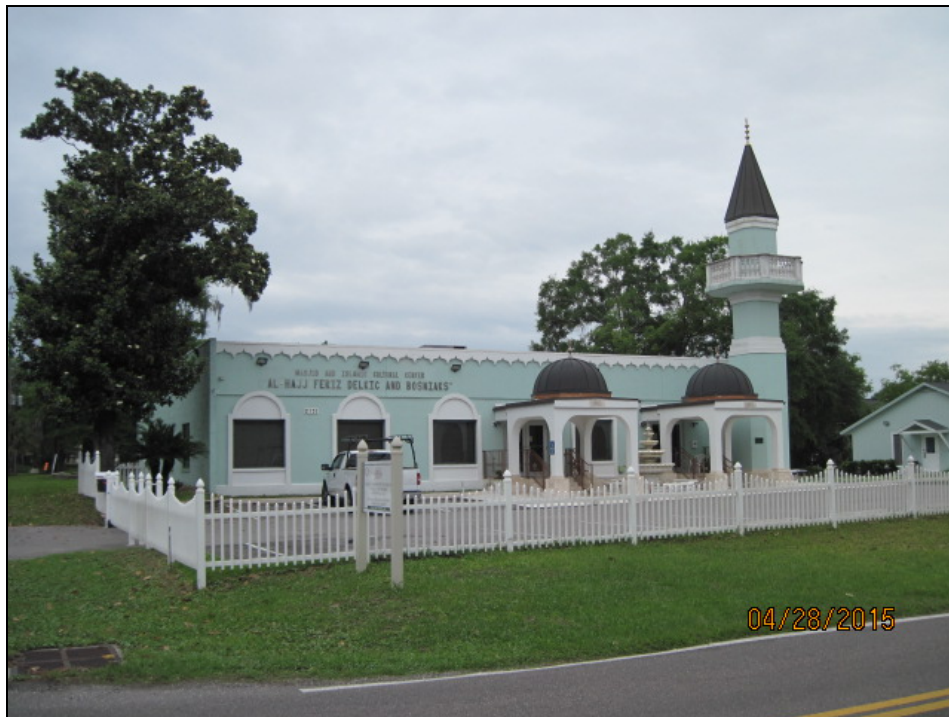
Mosque facility, 2131 Art Museum Drive
